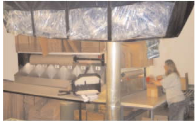
Custom overhead delivery system
