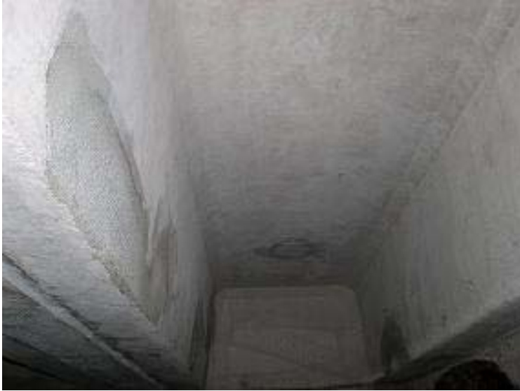
Figure 3.: Reprofiling concrete surface
