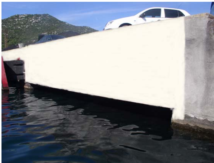
Figure 4.: MCI coating on the concrete surface
