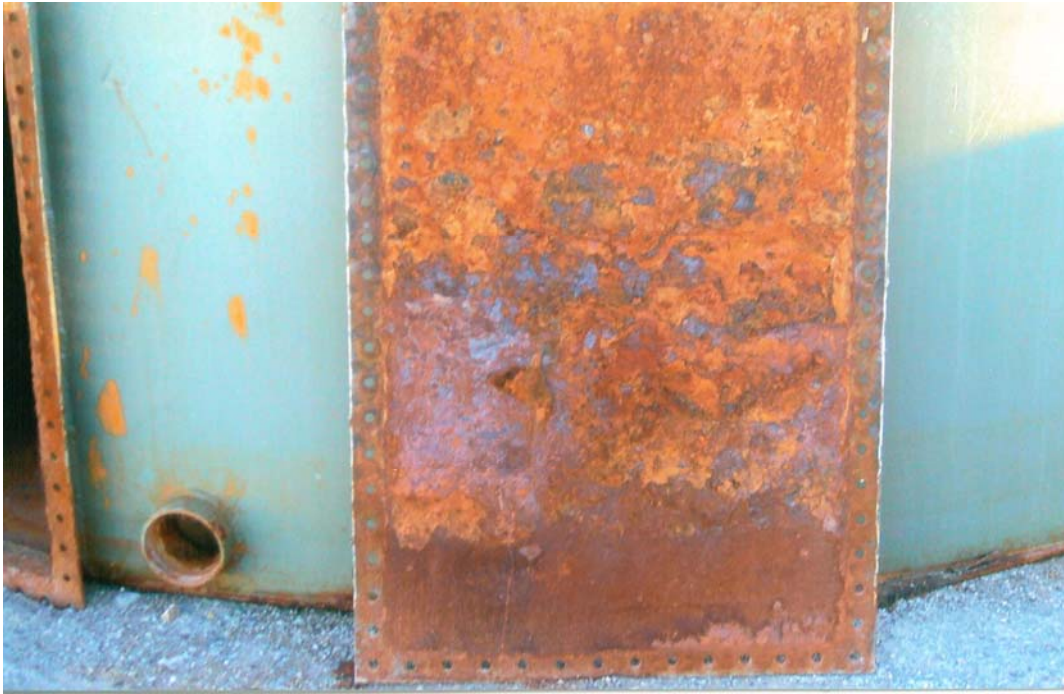
FIGURE 7 – Uncoated Holding Tank Hatch
