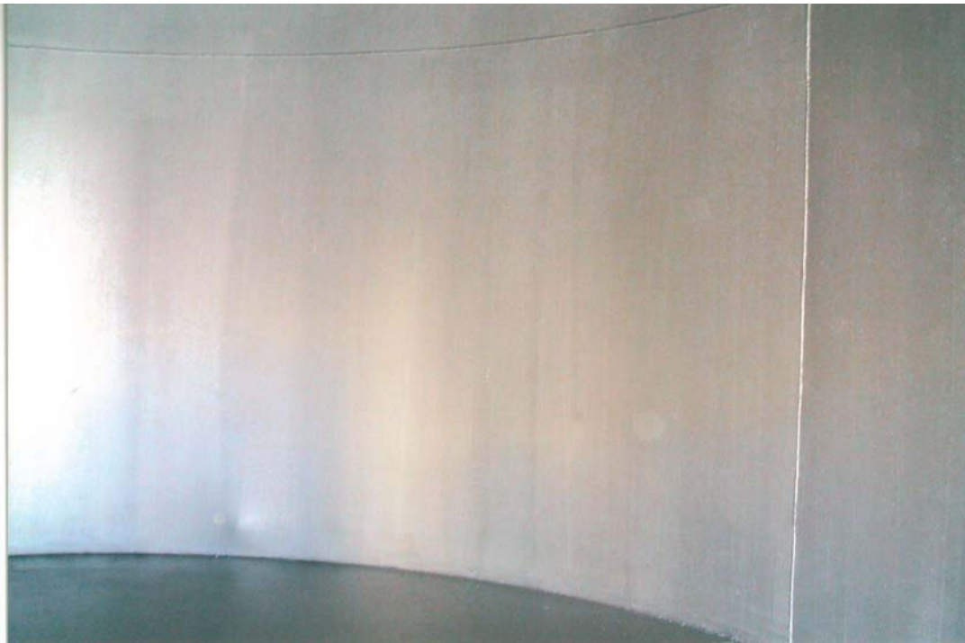
FIGURE 8 - Inside of Coated Tank
