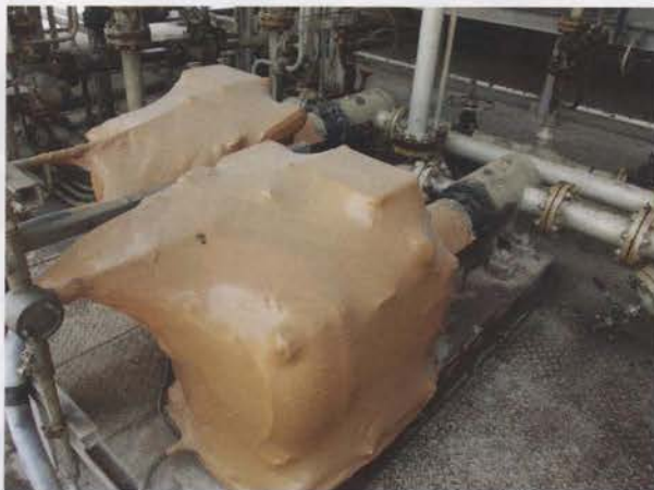
Figure 4. Equipment protected with MilCorr® film.
