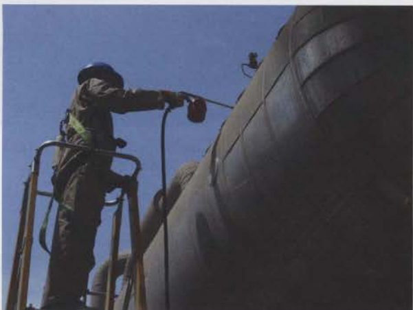
Figure 5. Insulated pipes being injected with VpCI® inhibitor.
