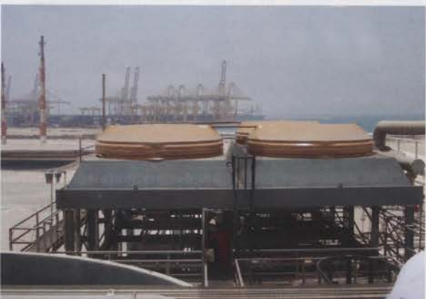
Figure 2. The fin fans were coated with Cortec coatings and covered with anti-corrosion MilCorr® film.
