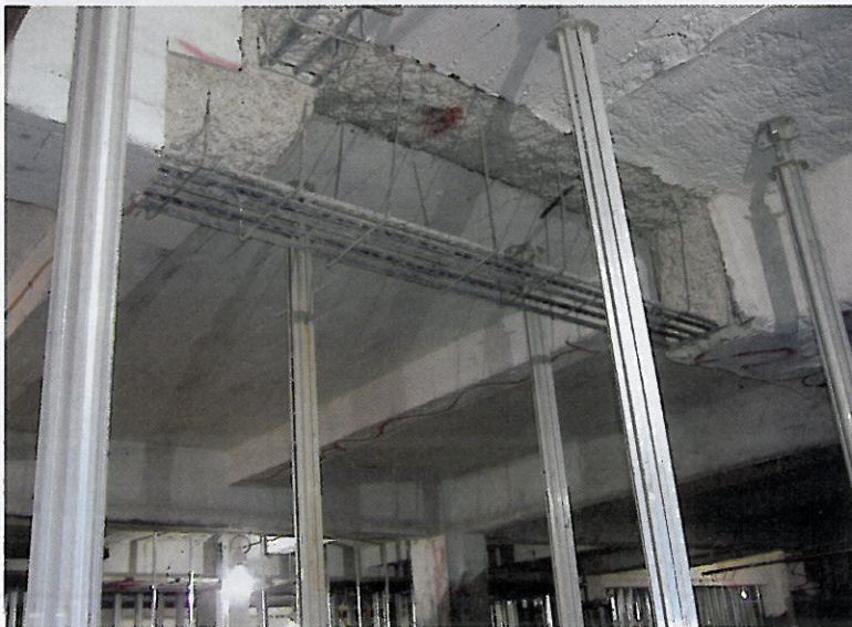
Interior beam repair work—notice the extensive shoring
