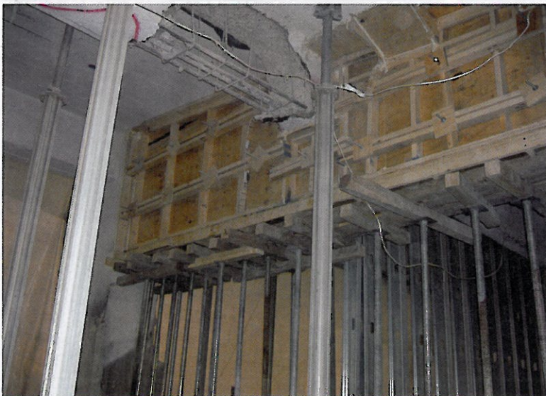
View of the full-depth beam repair
