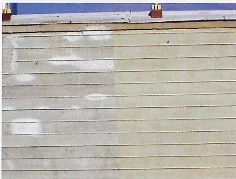
Before and after coating application
