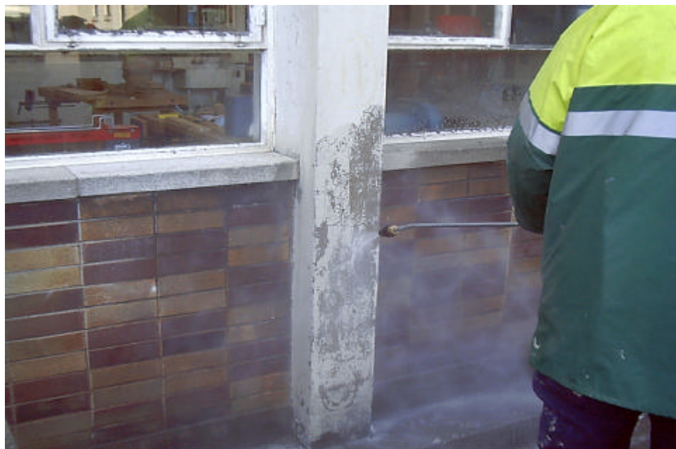
Figure 4: Surface Preparation by Water Jetting
