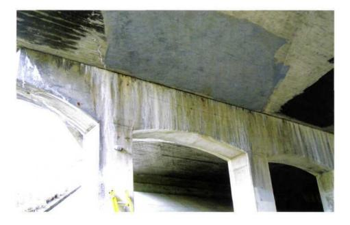
The GalvaCorr™ liquid coating is applied to concrete structures such as this bridge in order to protect the structures from corrosion.
