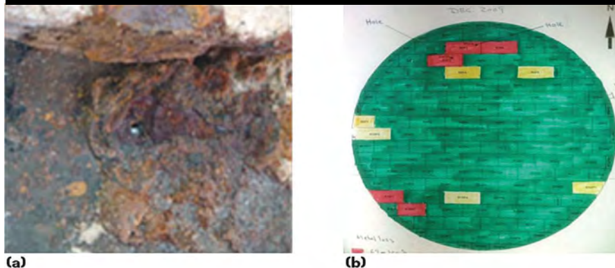
Bottom inspection Tank S-2 at South Terminal. (a) Penetration of bottom plate and (b) 2009 MFL test result.
