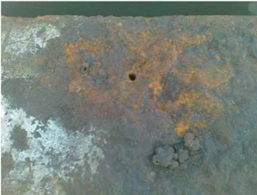
Soil-side corrosion on pilot project floor plate.
