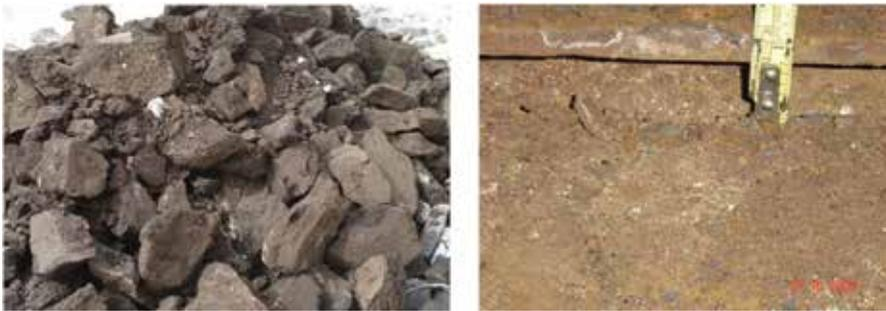
Oily sand excavated from below floor plates; air gaps of 5 to 50 mm under floor plates.
