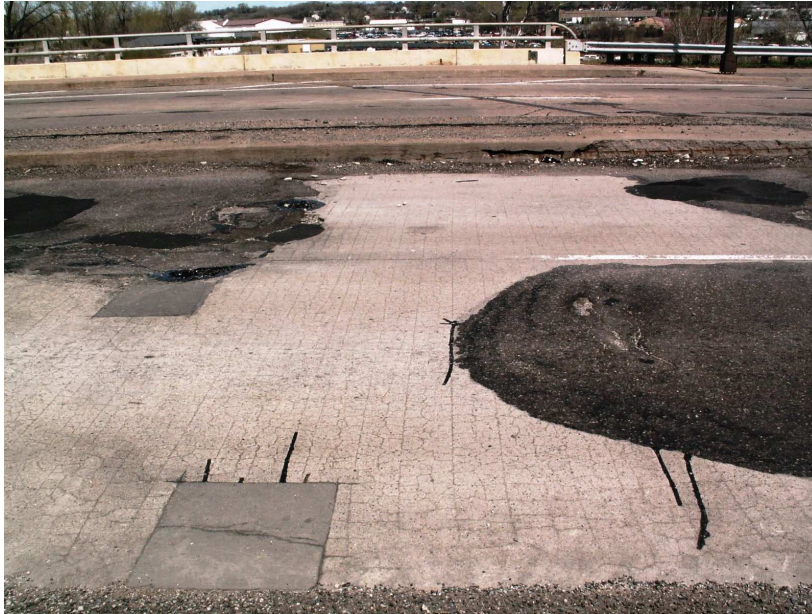
Figure 6 - View of Bridge Deck in 2007
