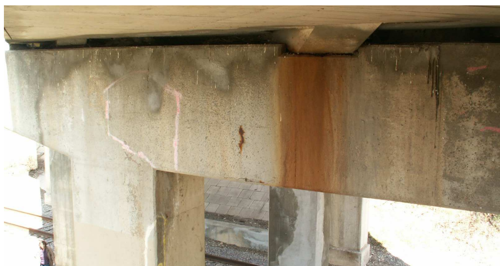
Figure 8 - Bridge piers without Galvanic Coating 4/2007
