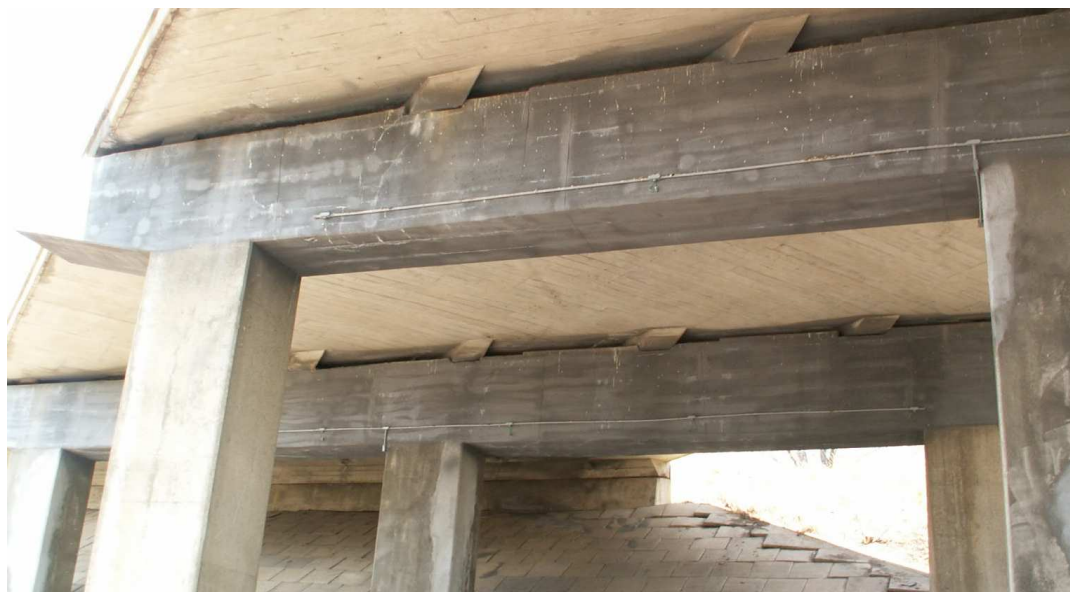
Figure 7 - Bridge piers with Galvanic Coating 4/2007
