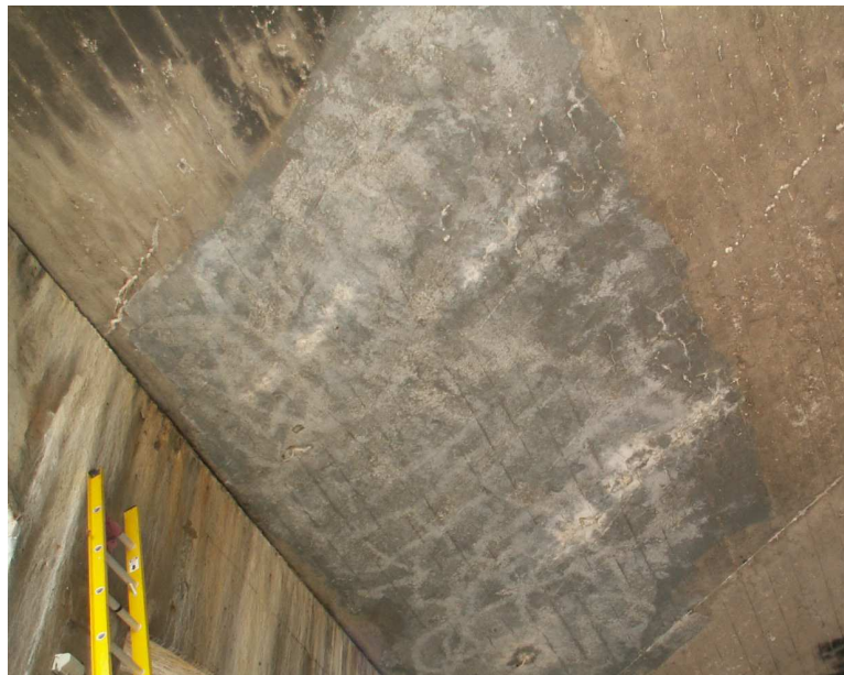
Figure 5 - View of Galvanic Coating under deck in 2007
