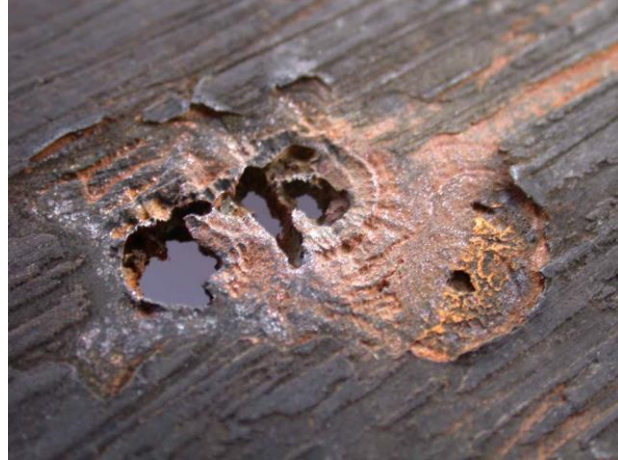
Pitting Corrosion on the un-protected tank bottom
