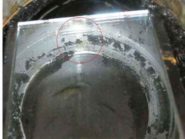
Nov 16: Corrosion on the seat pocket
