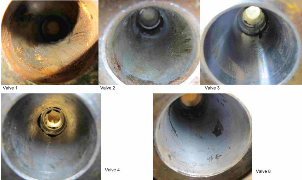
Figure 8: Pictures of the bore of each valve protected with water based inhibitor after the test was completed December 14 th .
