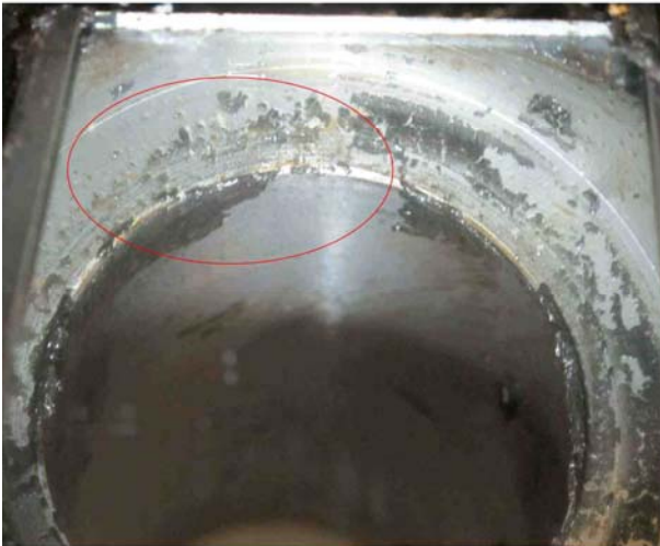
Nov 30: The corrosion can be seen developing at the top of the picture. (the bottom of the seat pocket)
