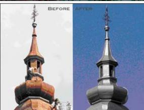
VpCI®-386 forms a fast-drying, thixotropic coating that is resistant to sagging or running, forming a tough, non-flammable protective barrier against corrosive elements. Its UV resistance and thermal stability gives outstanding outdoor corrosion protection without cracking or chipping with prolonged exposure to sunlight. VpCI®-386 can provide long-term protection for carbon steel, aluminum, stainless steel, galvanized steel, and copper.
