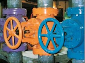
VpCI®-386 is a non-toxic, environmentally friendly, low VOC coating system, based on organic corrosion inhibitors. Cortec's proprietary organic Vapor phase Corrosion Inhibitors provide superior corrosion protection when tested against pigments and metal oxide based coatings. Applied, VpCI®-386 forms a protective film that is absorbed onto the metal surface, thus preventing corrosion.
