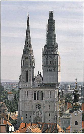
The neo-gothic towers of Zagreb Cathedral were restored using Cortec's CorrVerter. CorrVerter coating penetrated to the non-corroded part of the metal and stopped further advancement of the corrosion process.
