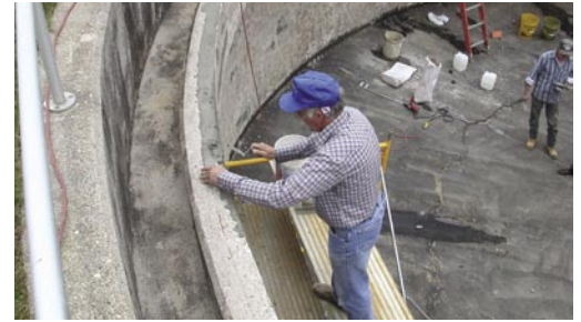
Waste Water Treatment Tank Restoration. MCI® 2020, 2023 & 2038.
