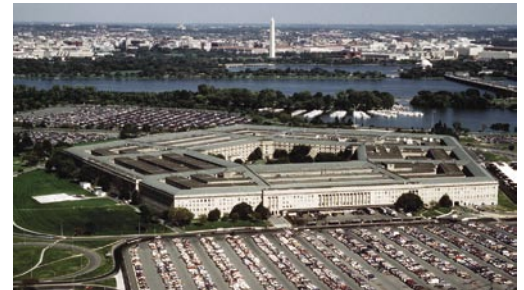
Restoration of all the Pentagon's exterior walls. MCI® 2020 V/0
