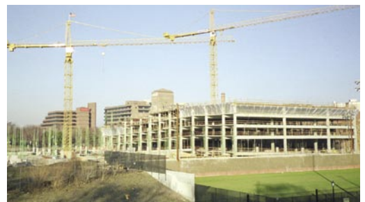
Construction of the Wells Fargo Parking Garage. MCI 2005® NS
