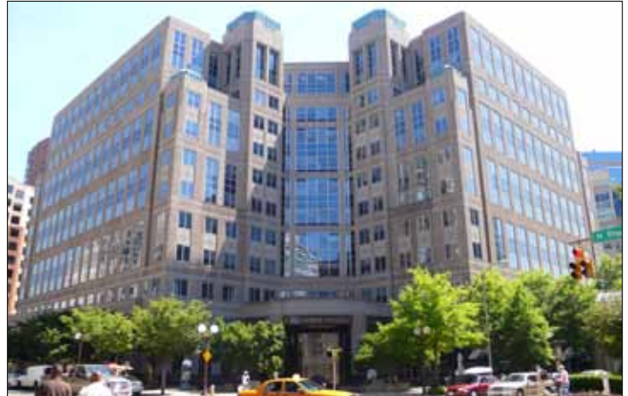
The National Science Foundation Headquarters located in Arlington, Virginia.
