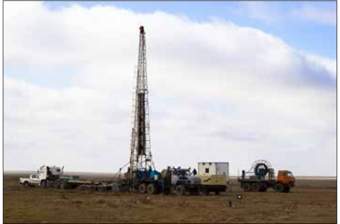
Drilling Tools Before Rust Removal
