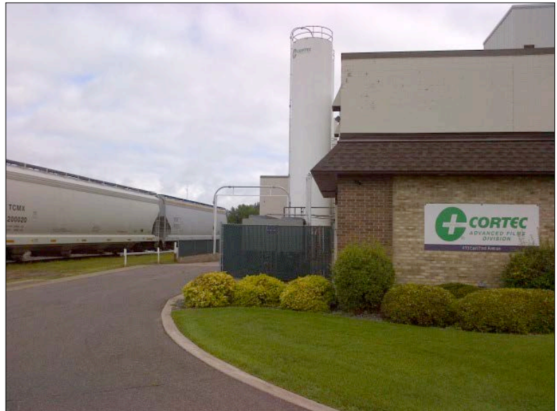
CAF receives its raw materials in rail car quantities making it more energy efficient, further reducing carbon footprint and lowering overall cost of production.
