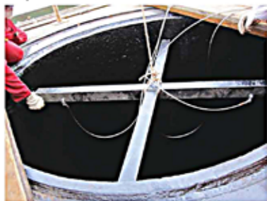
Steel frame setup for suspending VCI pouches.
