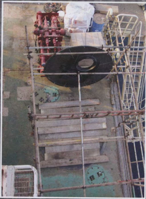
Main picture: Inside the caisson leg
