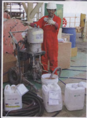
Top Right: Application of VpCI-609 S biodegradable powder using a pipe
