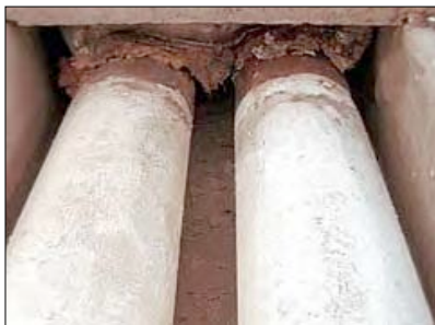
Corrosion under insulation (CUI)
