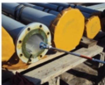
The VpCI®-337 fogging a pipe before capping.
