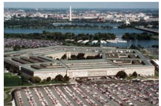
MCI 2020 will repair 200,000 square feet, and an additional 1,000,000 square feet of wall surface will be treated with MCI 2020 V/O.
