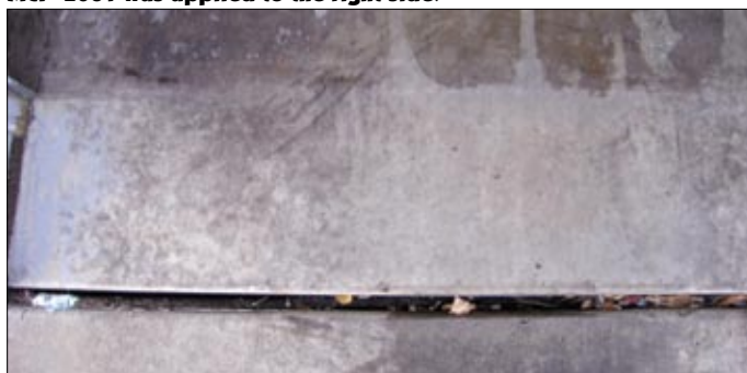
2. Garage doorway 12 hours after cleaning; MCI ® -2061 was applied to the right side.
