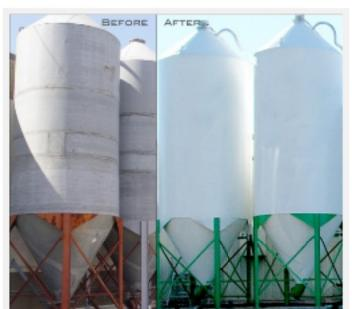
Cortec Corporation has introduced VpCI-386, an organic water-based acrylic coating that provides a multimetal corrosion protection in harsh, outdoor, unsheltered applications. Since it can be used as a direct-to-metal coating or as a finish coat, it reduces costs associated with corrosion said the company.
