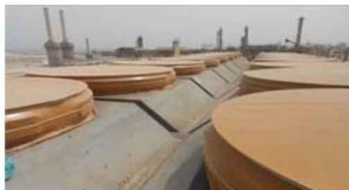
Photo: The fin fans were coated with Cortec® coatings and covered with anti-corrosion MilCorr® film (left). Equipment protected with MilCorr® film (right).
