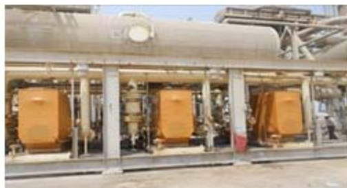
Photo: Mothballing of gas compressors and pumps (left). Insulated pipes being injected with VpCI® inhibitor (right).
