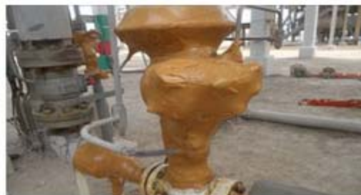
Photo: The fin fans were coated with Cortec® coatings and covered with anti-corrosion MilCorr® film (left). Equipment protected with MilCorr® film (right).
