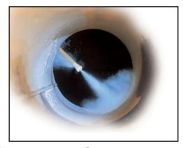
Fogging Cortec MCI<sup>®</sup>-309 Powder into girders provides immediate corrosion protection to the interior of box girders. No rinsing required before grouting.
