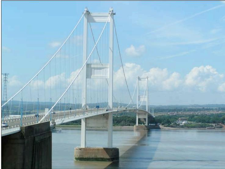
The Severn Bridge, in Wales, England, is a cable stay bridge maintained by the UK Highways Agency, and is an example of a bridge using this technology. The suspension cables on this bridge type are known to corrode over a long period of time. The first inspection of the main cables found they were corroded and had reduced structural strength. An acoustic monitoring
