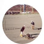
The concrete set up so uniformly, finishing, float work and brooming operations were completed on one end of a deck while pouring continued on the other end. Even with the low water content, the mix exhibited excellent finishing properties and the need for an evaporation surface retardant was very minimal.
