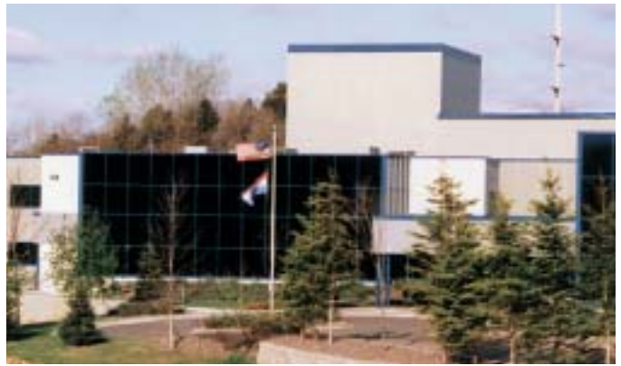
Cortec® Corporation's® World Headquarters in St. Paul, MN
