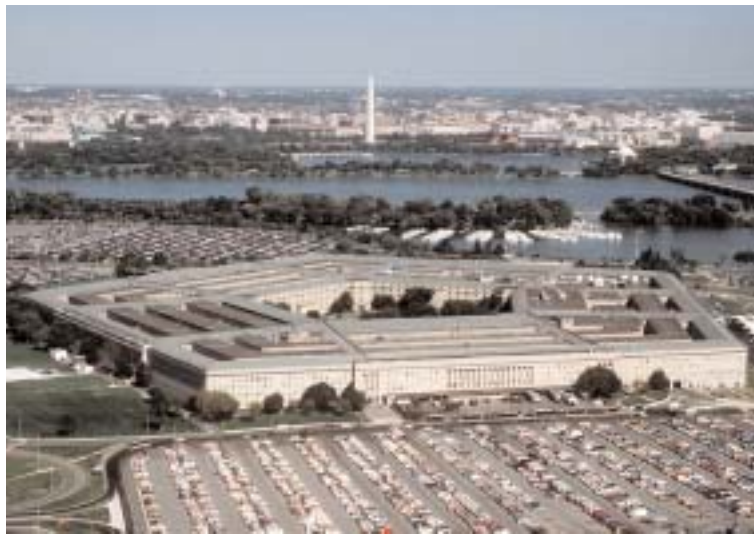
MCI 2020 will prevent corrosion at the Pentagon
