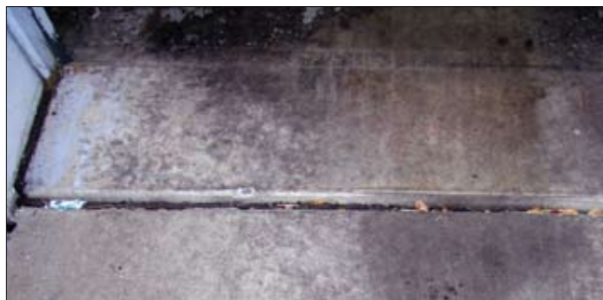
Garage floor doorway before the application of MCI®-2061.
