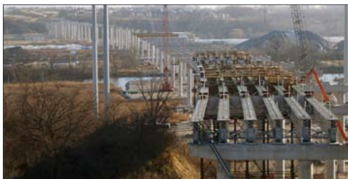
Des Plaines River Bridge
