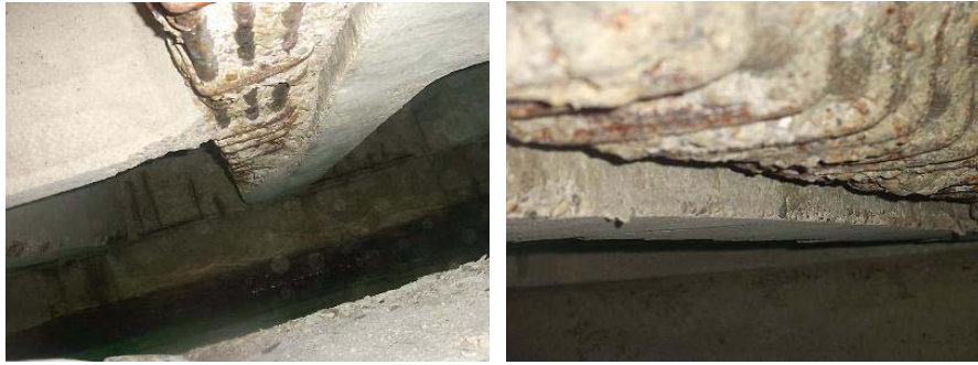
Figure 2.: Impregnation concrete surface
