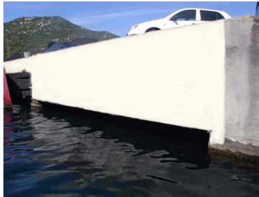
Figure 4.: MCI coating on the concrete surface
