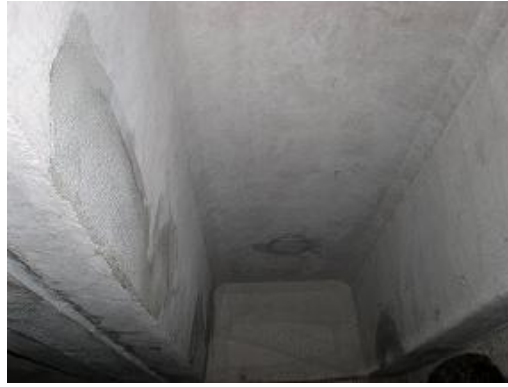
Figure 3.: Reprofiling concrete surface
