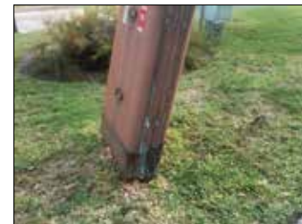
Corroded telecommunications enclosure packed with electronics ready to collapse.
