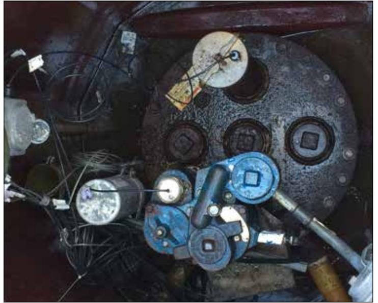
Cleaned, coated, and VpCI® treated sump at first station.
