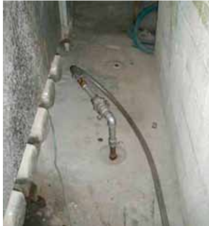
Injection of a remedial solution to decontaminate the soil.
