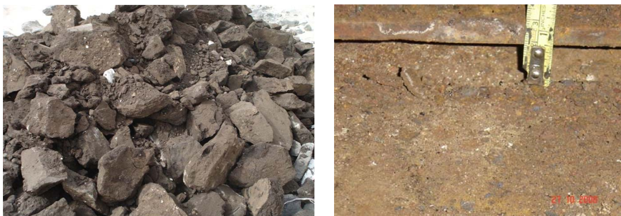
Figure 1: Oily sand excavated from below floor plates; air gaps (5-50 mm) under floor plates.
