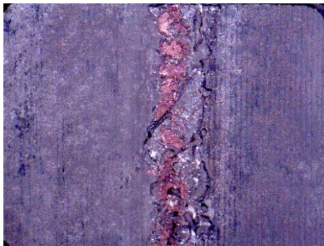
Figure 3. Traces of copper left on internal pipeline weld.
