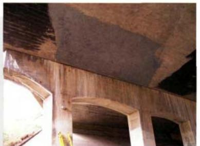
power washing the surface, at low ambient temperatures with good adhesion. If applied to a surface such as the underside or side of a structure, a top coating is unnecessary, but if applied to the top, a traffic-bearing coating is needed. The fast-acting coating also offers 5 to 7 years of cathodic protection.
