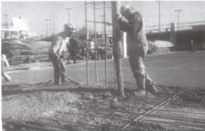
E-Con-Placer's president, Rob Tousignant, said the concrete mix enabled his firm to pump at lower pressures, providing a productivity increase.
