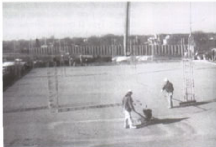
Concrete pumping company E-Con-Placer reported that the pioneering mix, while low in water content, flowed easily and consistently.
