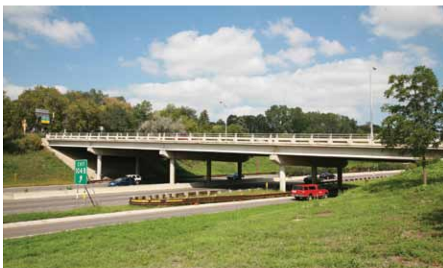
Constructed in the early 1960s, the Randolph Avenue Bridge in St. Paul, Minnesota, required extensive repairs from the results of chloride-induced corrosion of the reinforcing steel.
