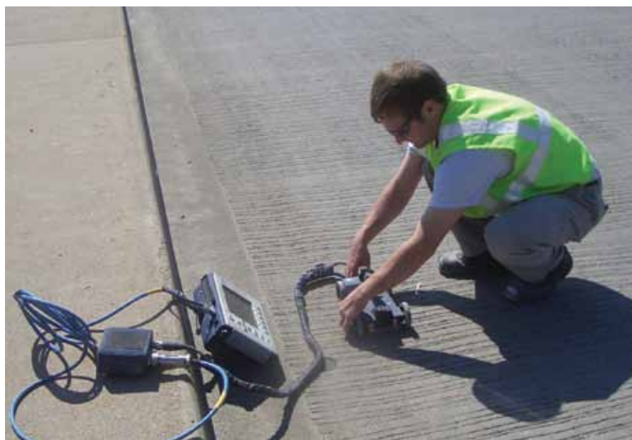
Ground-penetrating radar was used to locate reinforcing steel in the bridge.
