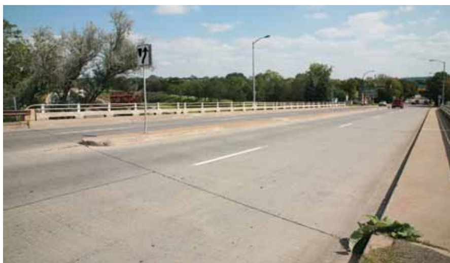
The westbound lanes of the Randolph Avenue Bridge were treated with a migrating corrosion inhibiting admixture and compared to the eastbound lanes that were refurbished with an untreated concrete overlay.
