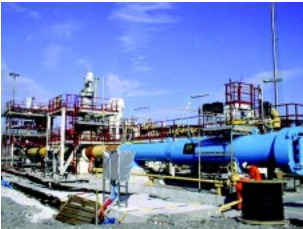
Pig-launching installation.
