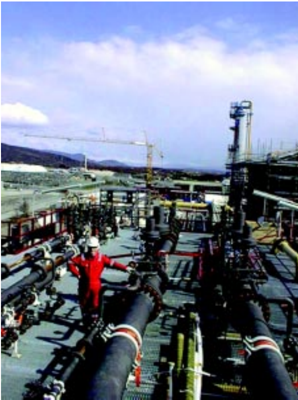
Onshore pipeline installation.
