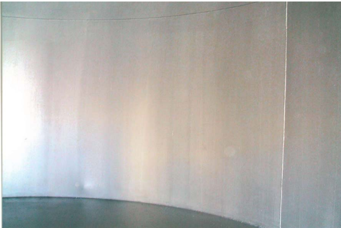
FIGURE 8 - Inside of Coated Tank
