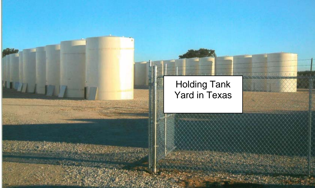
FIGURE 5 - Holding Tank Yard in Texas
