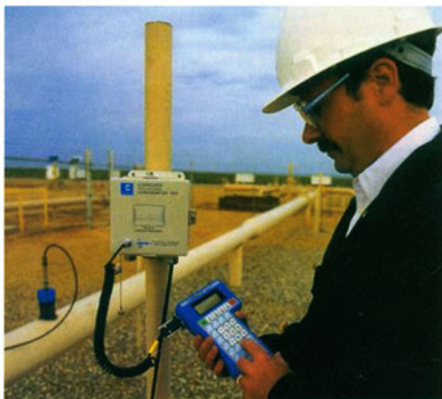
Corrosion probe connected to a remote data collector. The data are being transferred to a handheld data logger.
