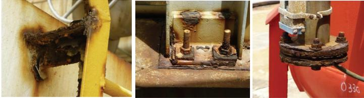
Typical appearance of degraded coating on a badly maintained 'aged' industrial structures.
