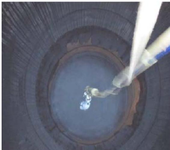
**Figure 2: Application of Inhibitor A using a pipe coater**
