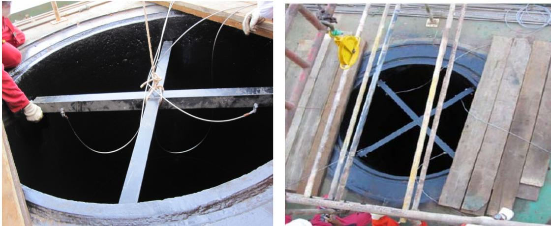
**Figure 3: Steel frame setup for suspending Inhibitor B pouches.**
