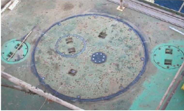
**Figure 5: Caisson Leg Sealed Cover**
