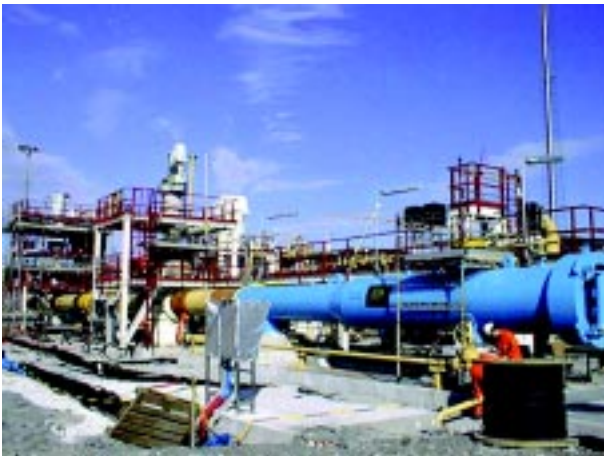
Pig-launching installation.
