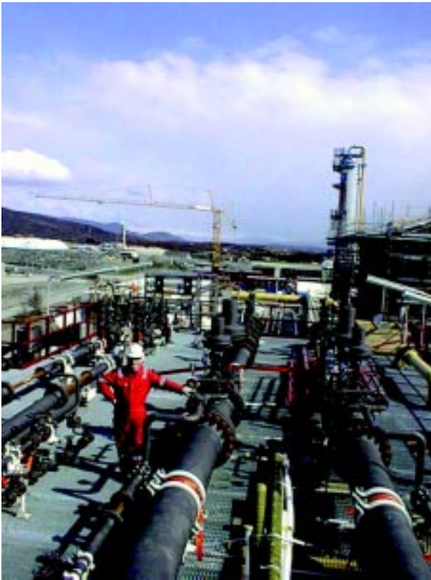
Onshore pipeline installation.
