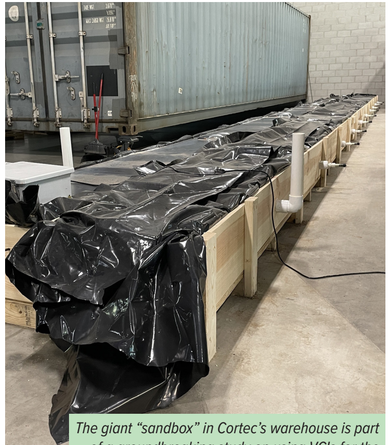
Applying VCI to the sand test pad, aka, the Cortec® “sandbox.”
