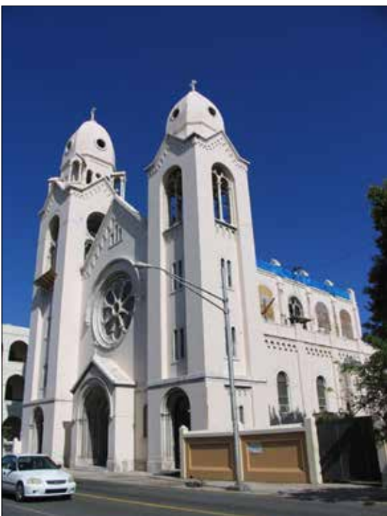
Case History #349: "Repair of San Agustin Church"
