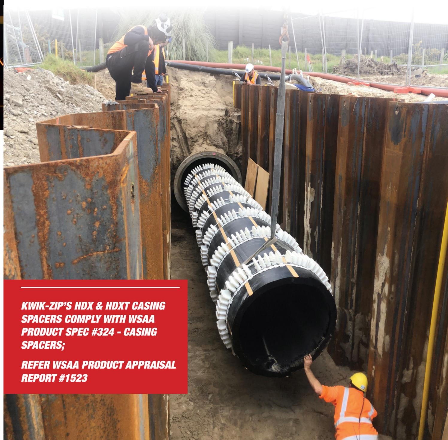
**KWIK-ZIP'S HDX & HDXT CASING SPACERS COMPLY WITH WSAA PRODUCT SPEC #324 - CASING SPACERS;**
